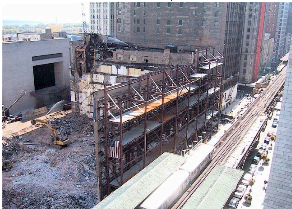
Wabash Wall Structure Being Supported
