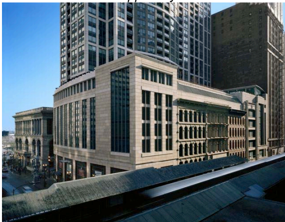
Completed Restored Wabash Facade
